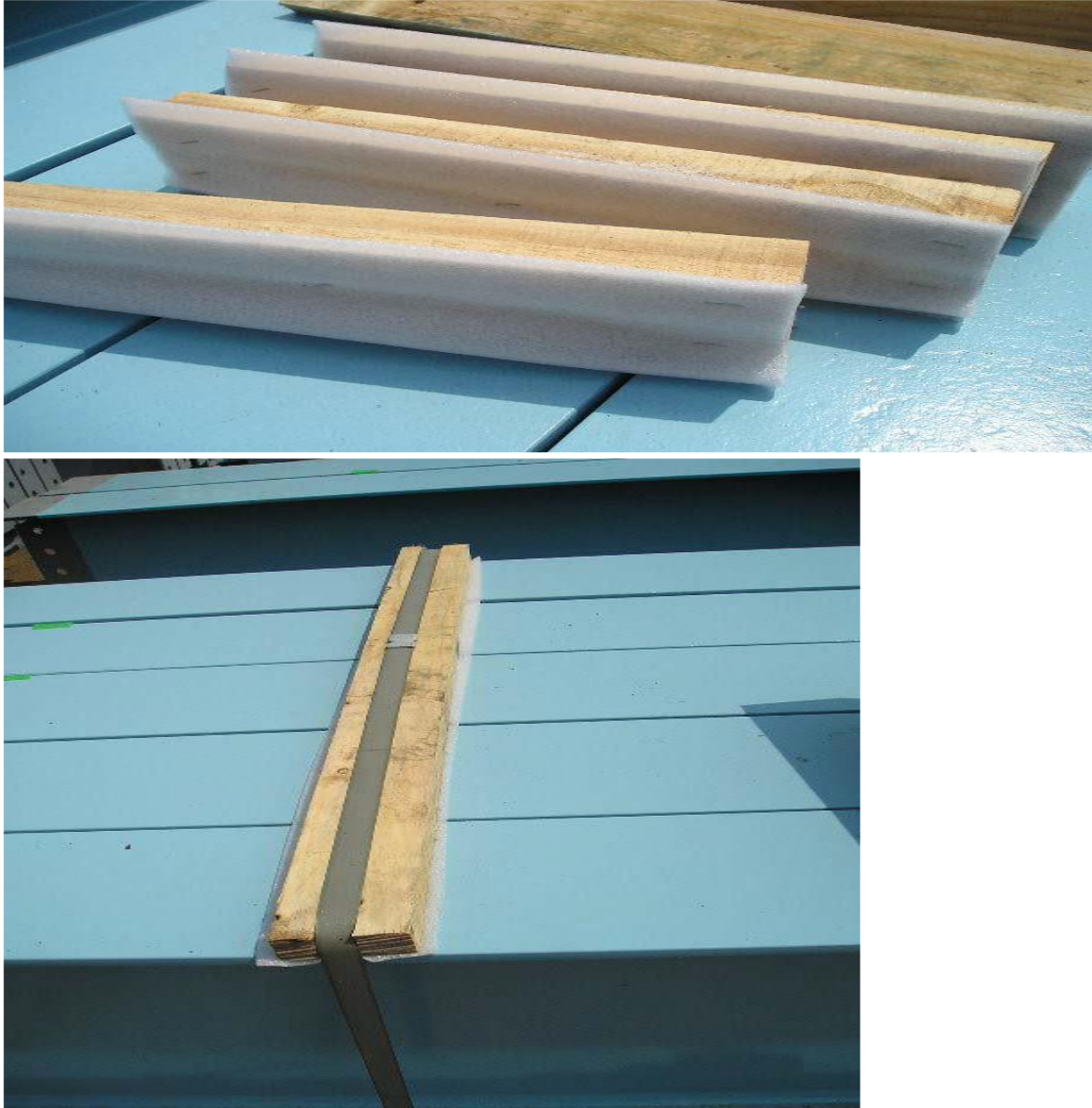
Figure 6. Preventing painting damage
