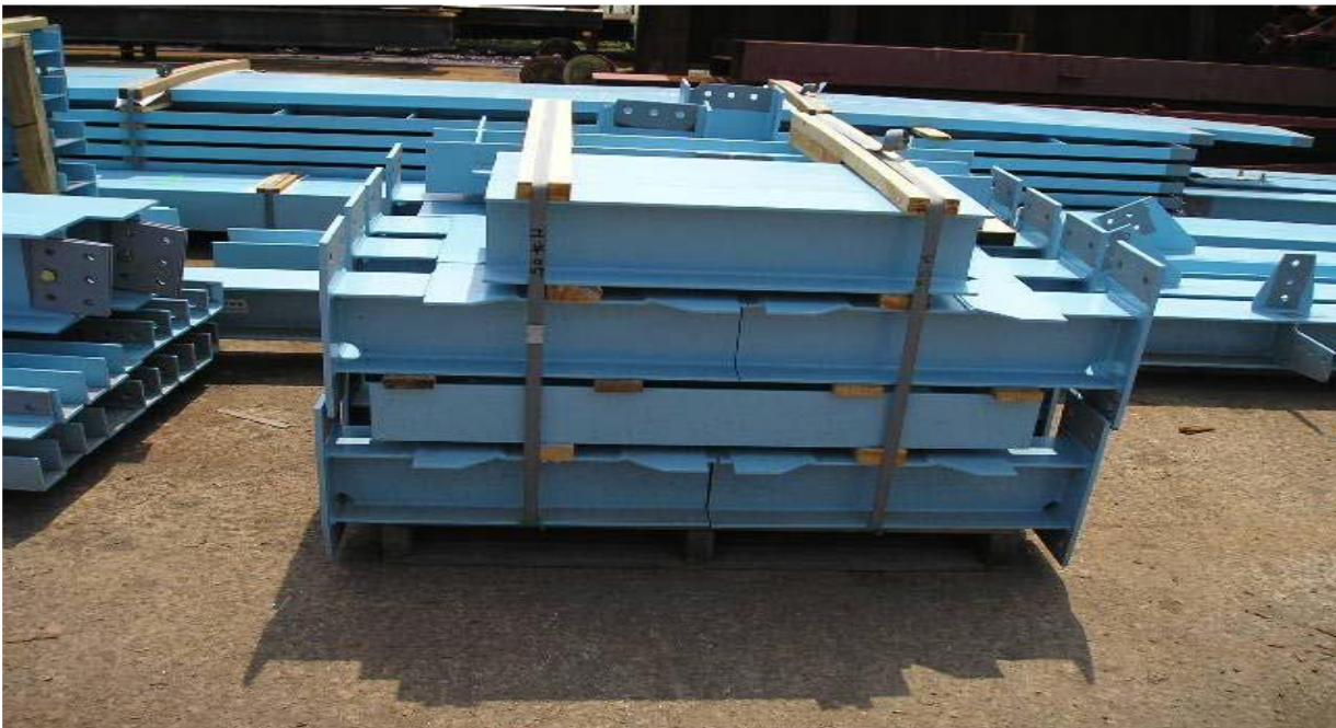
Figure 5. Using thin timber between items
